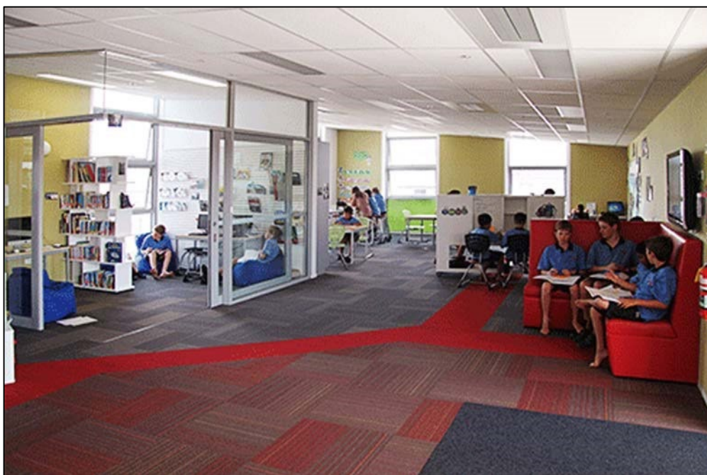
Figure 19: Side Lighting Design Principles – tall windows in more than one wall, with borrowed light via glazed walls to break out/study space
