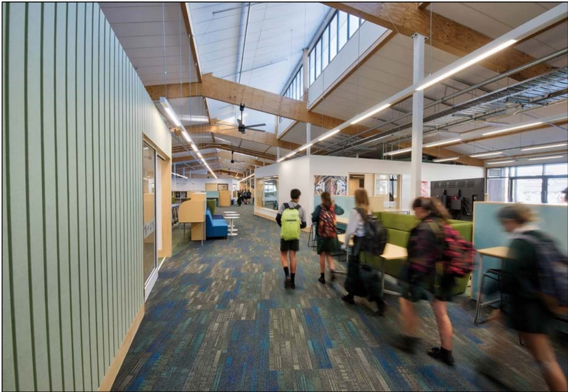
Figure 22: High ceiling and central clerestory rooflight.
