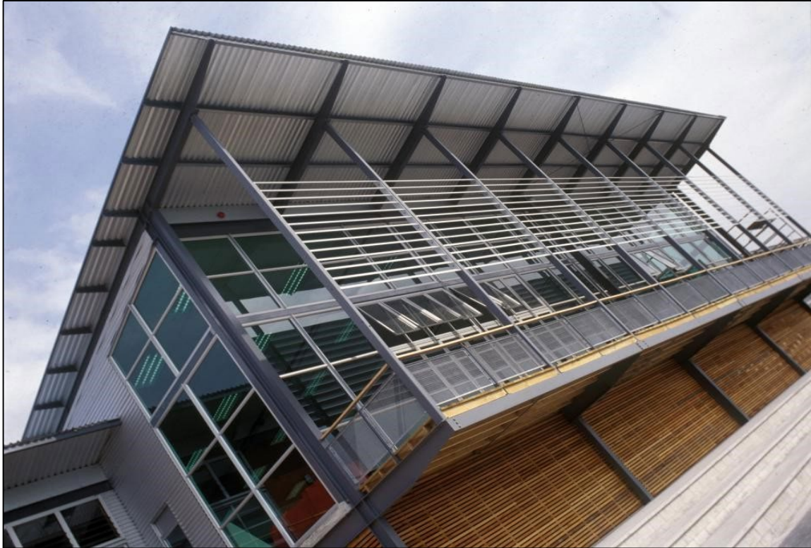
Figure 16: Combination of sunscreens and overhangs provide a good level of solar shading and daylighting
