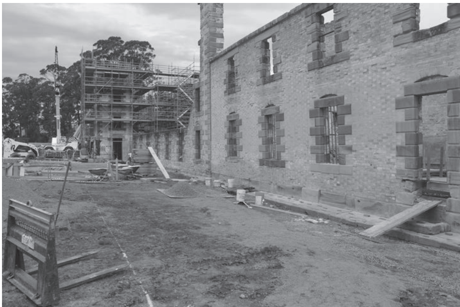
Figure 0.8 Photo taken from the muster ground during conservation works in 2015. (PAHSMA 2015)
