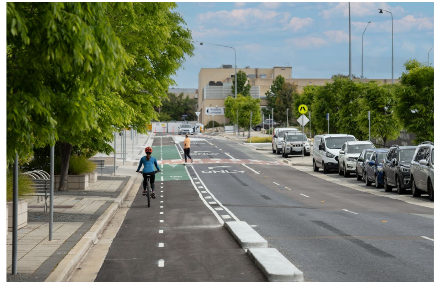
Figure 6. Example of a town centre collector/ Vibrant Street including a clear footway, furniture zone with plantings, protected cycleway at road level (two-way), raised pedestrian crossing, indented on-street parking and castellated buffer. (Furzer Street, Phillip).
