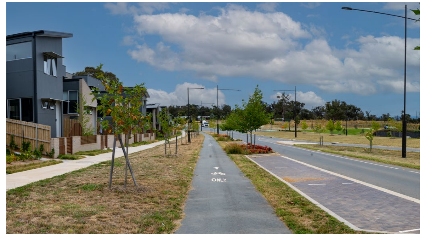
Figure 5. Example of a movement corridor / suburban arterial cross-section including a footpath, protected cycleway at verge level (one-way), street trees, landscaped buffer and indented on-street parking and roadway with a median. (Pro Hart Avenue, Strathnairn).
