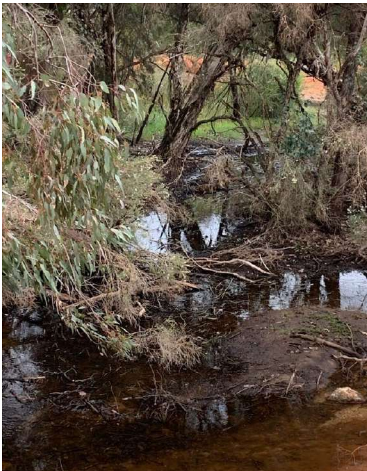
Photograph 3: Thirty-Four Mile Brook Culvert Location Looking Northeast Towards Existing Crossing
