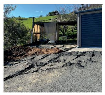
The photo shows a buckle in the asphalt surface at the bottom of a hill, indicating the potential for a slumping failure along the slope and the possibility of more slips in the future.
