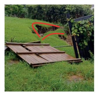
The photo shows the formation of a head scarp\* and land slicing, indicating a slumping slope failure with potential for further slips. The base of the failure may show bulging of the land. The damage also reveals tilting and displacement of the fence.
