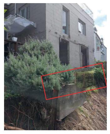
The photo shows a landslip below a building. Horizontal support to the retaining wall immediately below the building has been compromised. The foundation of the concrete wall has lost support and further failure is likely to occur soon.
