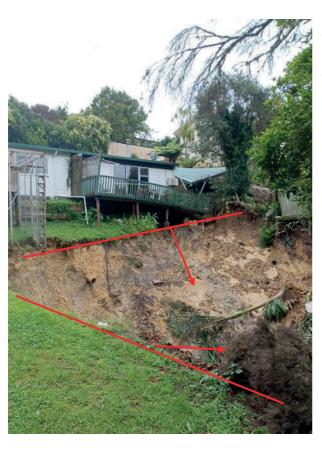
A landslip has occurred below a building and a carport. This photo shows an evacuation of soil, and damage to the buildings, including loss of vertical and lateral support to the corner deck piles. The carport structure has visibly slumped. Lateral support to the foundations needs to be considered.
