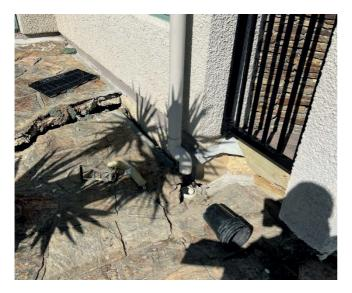
The photo shows a formed crack and an offset in the storm drainpipe. This indicates ground movement which may affect the building foundations and could be worsened by concentrated stormwater discharge into the displaced ground. Further movement may occur.
