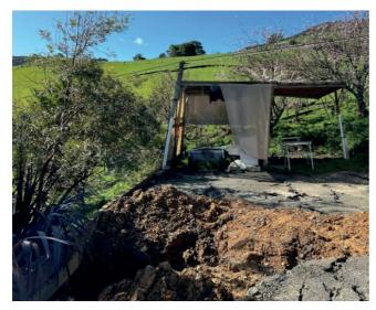
The photo provides a different view of a head scarp forming above the property. Combined with the buckling of surface asphalt seen in a previous photo, this suggests the instability may extend across the building platform.
