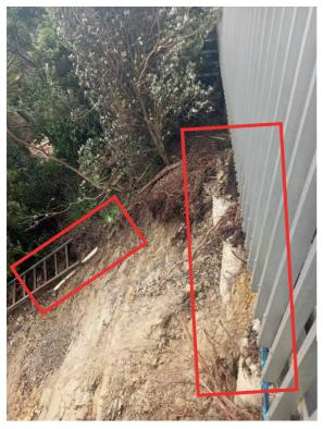
A shallow slip has exposed the foundations, as well as the once buried underground services. The soil around the front piles has been lost or reduced. The capacity of the deck to resist horizontal force may be compromised
