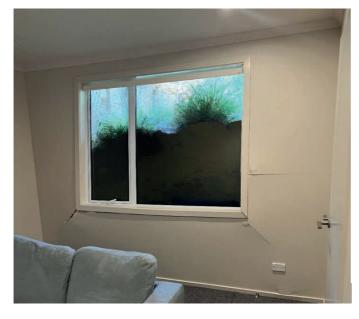
The strength of the external wall of the building has been significantly exceeded and has bulged inward. Internal linings have cracked and the horizontal strength of the building has been compromised.
