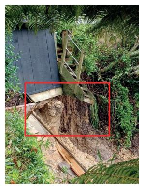
A slip has occurred. The foundations have been exposed and rotated which has compromised the building's structural integrity.
