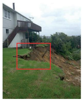
The photo shows the upper times decking has disconnected due to the land slip. Other piles also show signs of movement to varying degrees.
