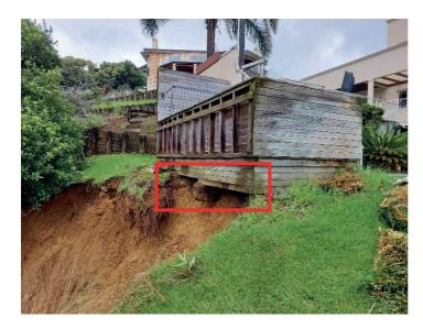
The landslide has exposed the concrete foundations. The supporting soil around and below the foundation has been lost. The loss of support is evidenced with sagging visible of the decking.
