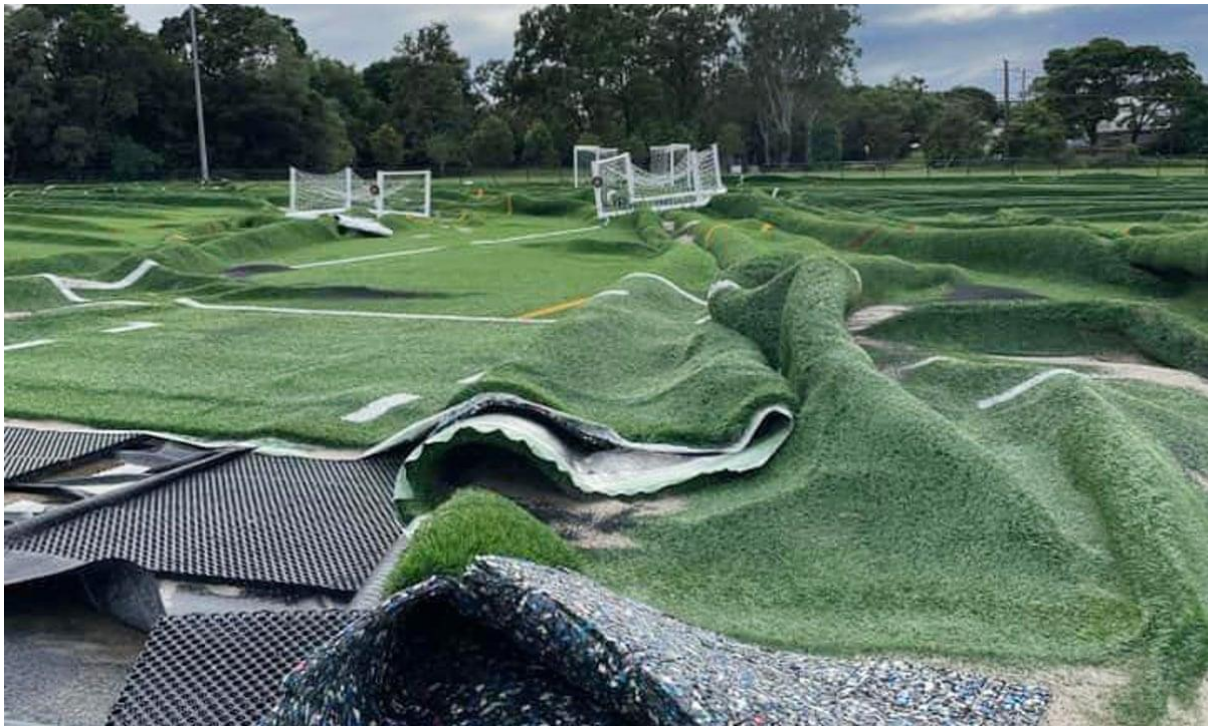
Figure 6: ST mat on a Brisbane field which was lifted during the March 2022 flooding [24]
