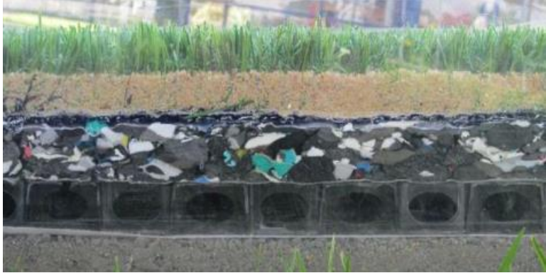
Figure 3: Cross section of a ST profile with horizontal drainage cells from Sheppard (2021)
