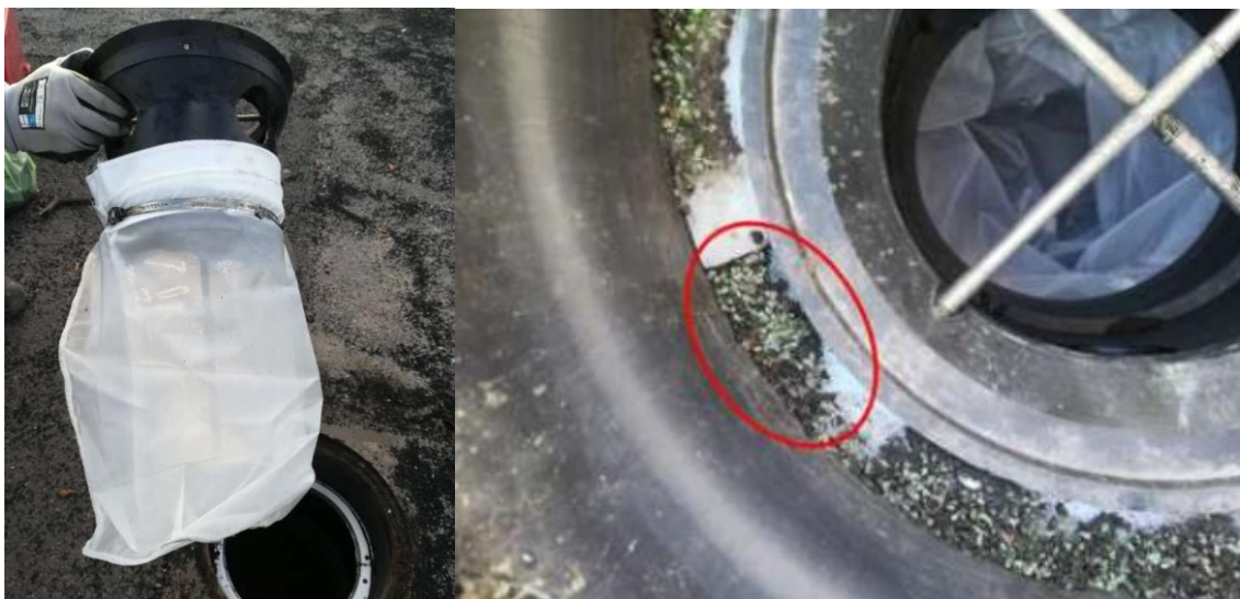
Figure 9: Example of a filter installed in drains surrounding ST fields to trap infill particles (left) and infill bypassing the filter where the seal is poor (right), from Lundström (2019)
