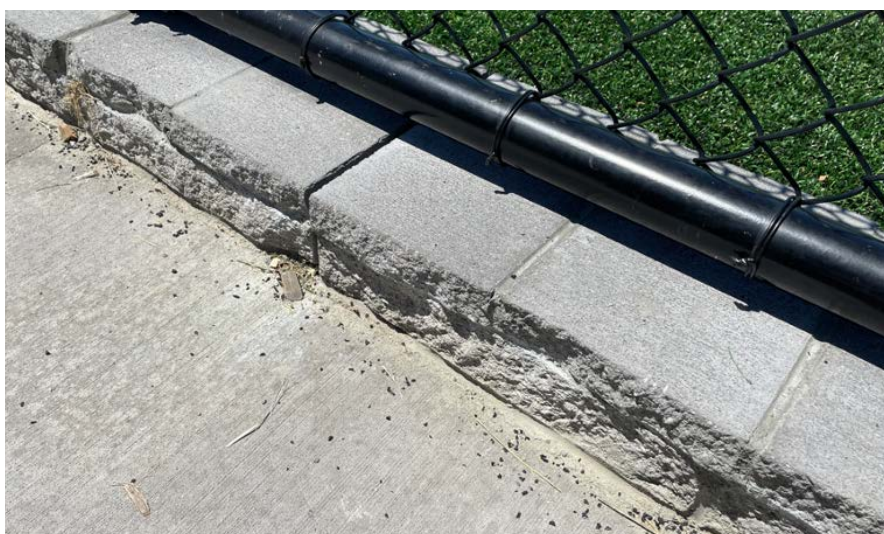
FIGURE 1: An example for tracking of rubber crumb infill from synthetic turf sport fields. The image was taken on 22 February 2022 at a recently opened soccer field in Sydney. The access gate to the field, equipped with a brush-gris system to collect crumbs was approximately 12 meters away from the section shown in this image..
