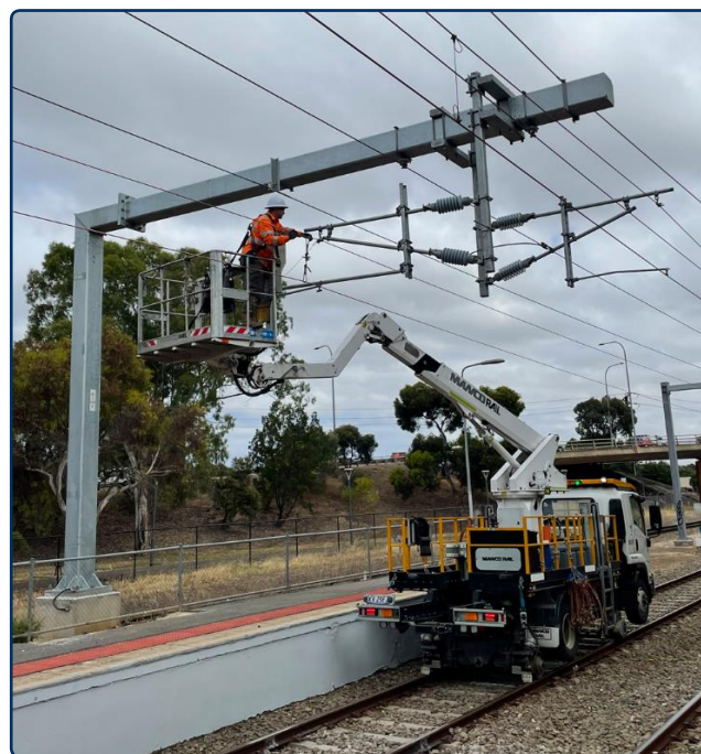
The final section of overhead wiring was installed on Friday, 14 January 2022
