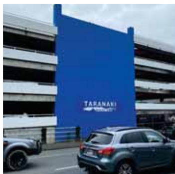
We allocated over $5m to earthquake strengthening the Downtown Carpark building so it can be re-opened for public use.
