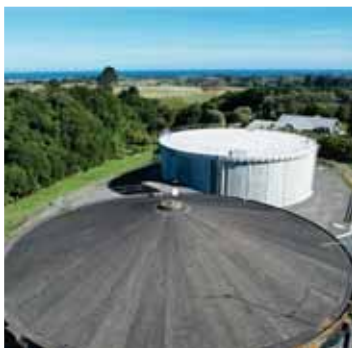
Two drinking water reservoirs, costing $18m, completed at Henwood and Mountain roads to supply Bell Block, Waitara, Lepperton and further north.
