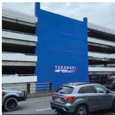
We allocated over $5m to earthquake strengthening the Downtown Carpark building so it can be re-opened for public use.
