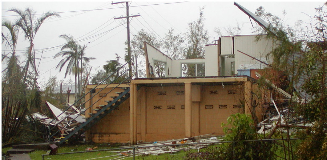
Inadequate tie-down through the entire structure.
