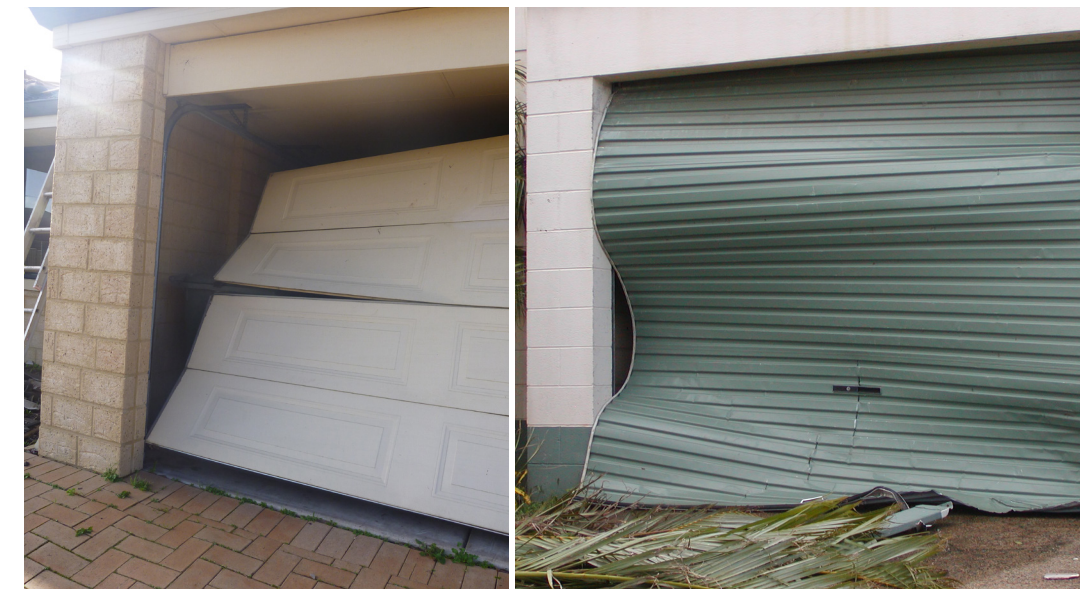
Cyclone damage to older garage doors
