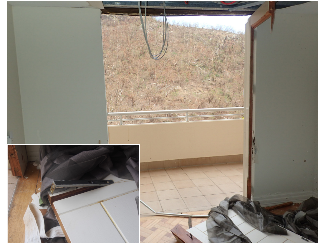
A door that had inadequate fixing to the wall frame and inadequate door latches
