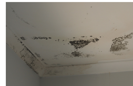
Mould on ceiling
