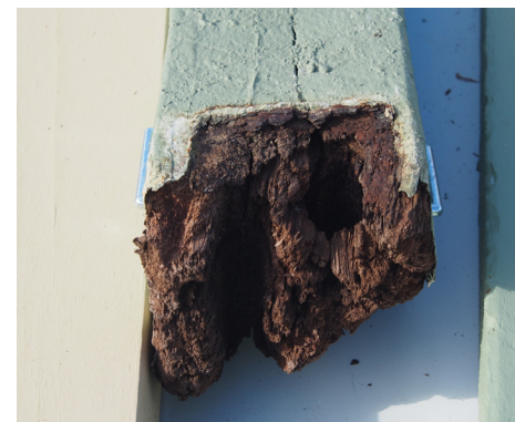
Rotten members such as this veranda post may fail under strong wind loads.
