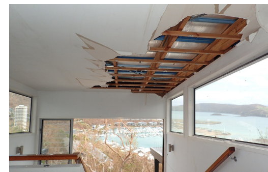
Damage to plasterboard ceiling
