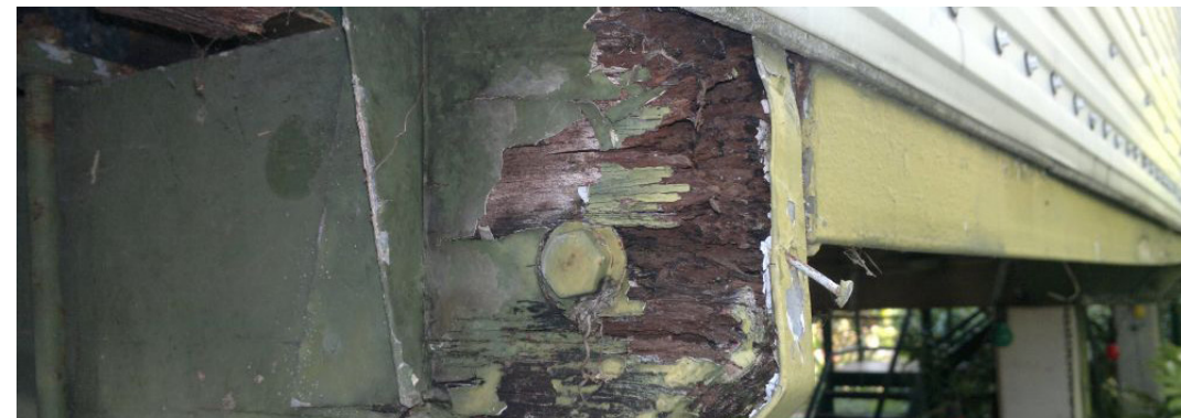
Rot in part of the sub-floor structure. The timber needs to be replaced, not just painted over.
