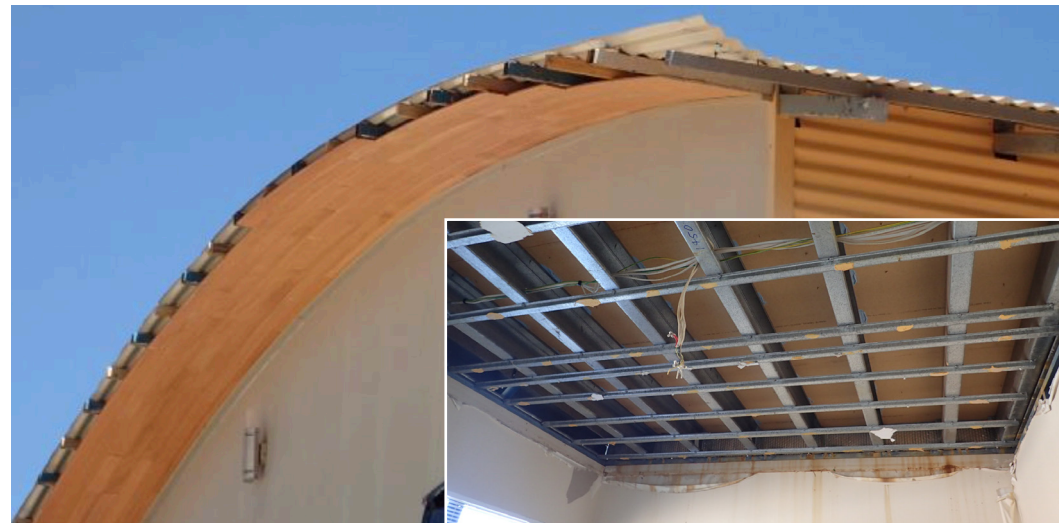
Damage to flashings (inset shows water damage to ceiling)
