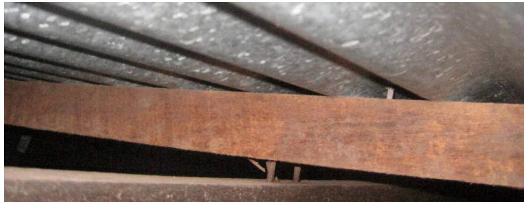
Partial failure of batten to rafter connections during a cyclone
