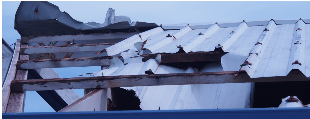
Roof loss caused by corroded roofing screws
